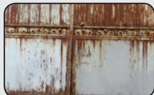
Ponçage 1er passage, gros grain 1st sanding passage, big grit
